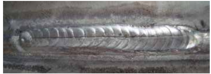
Cracked repair weld due to improperly preparing the repair area.
